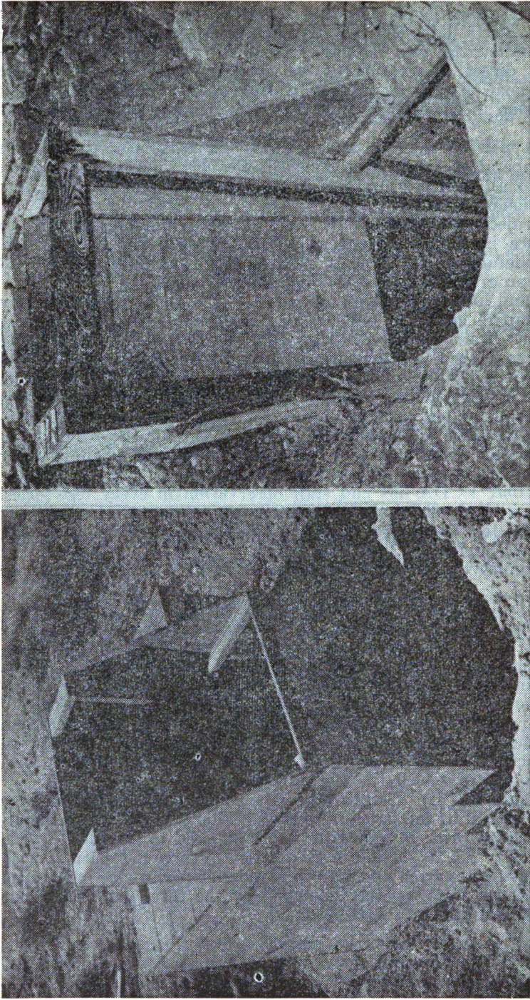
SLIDE No. 1.—Covered trench-type shelter.
